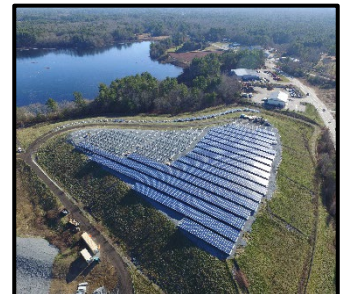
1.8 MW NORTH CAVER, MA
