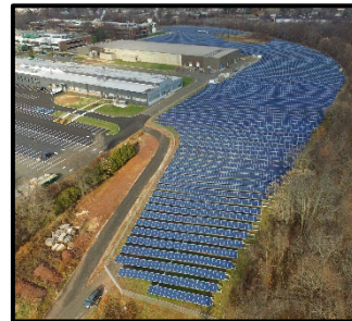
3.1 MW BRIDGEWATER, NJ
