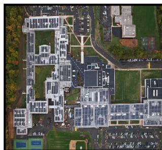
2.8 MW WARREN, NJ
