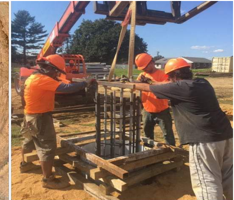
Placing Rebar Cages
