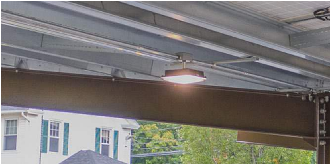
Figure 3. SMLLC LED Light suspended from an electrical work box, EMT and Uni-Strut
