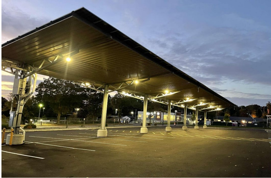
Figure 4. Lights mounted near the strut at the end of the Bay.
