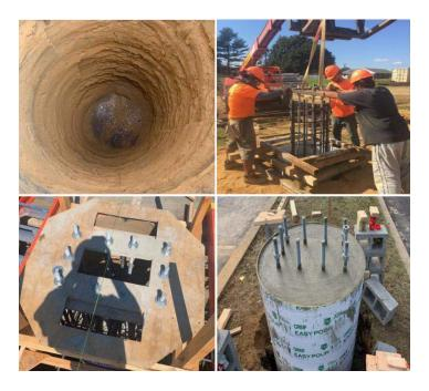
However, Spread Footings do not require as deep an excavation, requiring a much shorter concrete forming tube and flatter rebar mat with pier uprights in the center (see images below).
