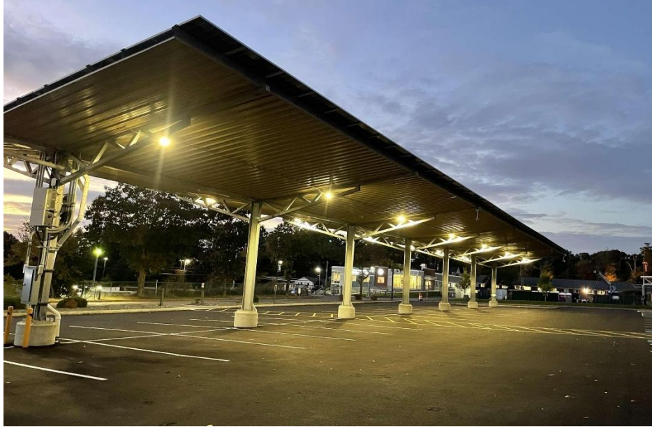
Figure 5. Lights mounted near the strut at the end of the Bay. Acceptable
