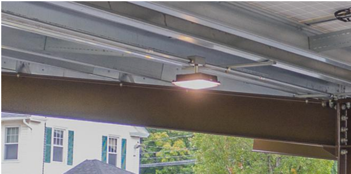
Figure 2. SMLLC LED Light suspended from an electrical work box, EMT and Uni-Strut
