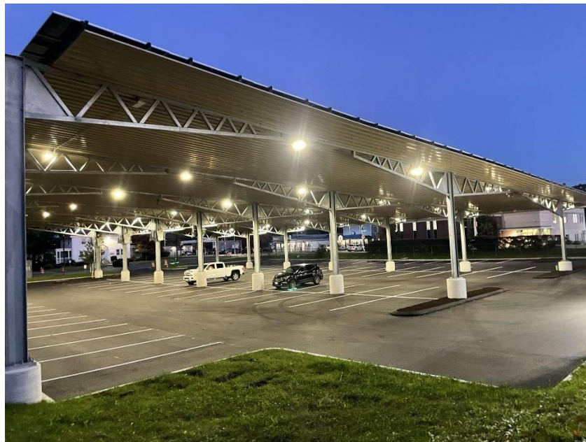
Figure 4. SMLLC lights mounted in the middle of the Bay by Solar-Construction
