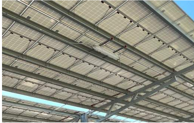
Figure 3. Contractor-supplied fixture fastened to the SMLLC purlins with Uni-Strut
