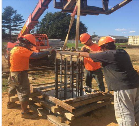
Placing Rebar Cages
