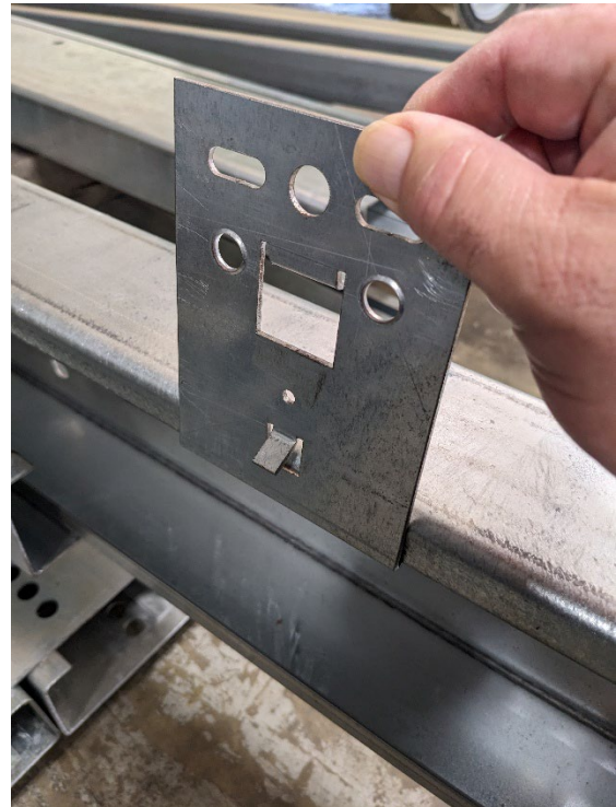
Panel Bracket hooked on C-Channel Purlin
