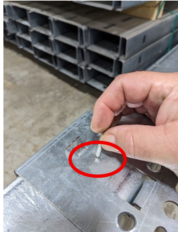
Alternate Panel Bracket Mounting Screw Position
