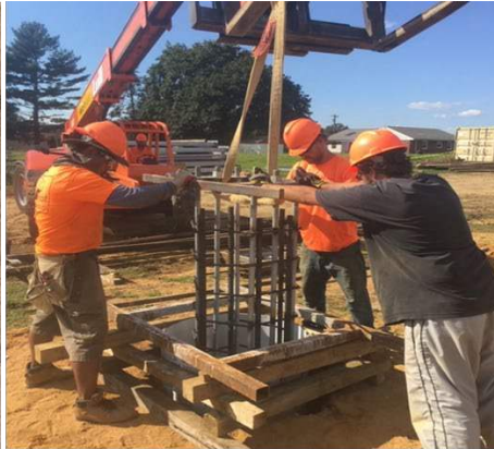
Placing Rebar Cages
